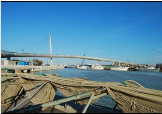
Figure 11. The bridge and the channel port (Source: E. Taglieri)
