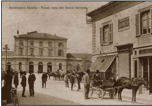
Figure 1. Castellammare station (1916) (Collection: R. D'Amario)
