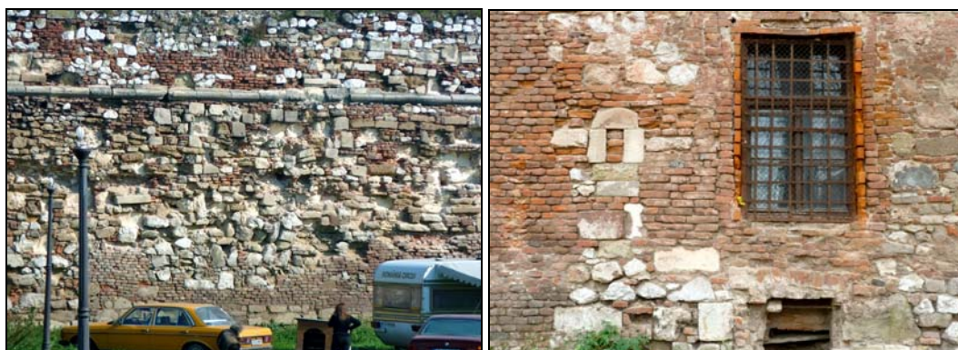
Figure 15. White limestone, probably from the Betfia quarry (left image) and fragments of the architectural and structural elements of the earlier Medieval fortress (right image) incorporated in the red-brick walls of the Renaissance fortress
