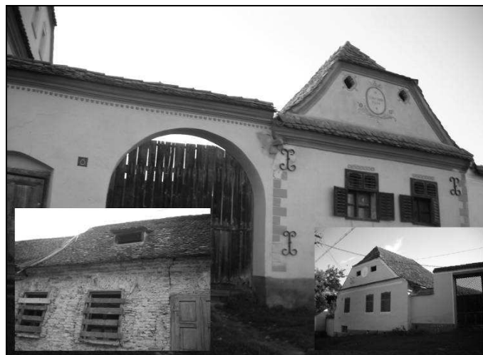
Figure 2. Viscri Village. Houses carefully rehabilitated only with traditional techniques and materials.
