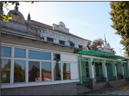
Figure 6. Baile 1 Mai. The former casino building
