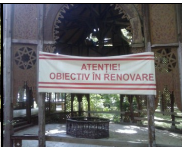
Figure 13: Restoration in progress in the central part of the Park
