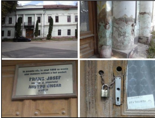
Figure 1. The former Royal Villa in Buziaș resort now derelict and locked
