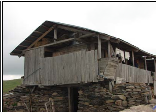
Figure 3. In some of the plateau houses in the field, used as an barns ground floors was built of stone
