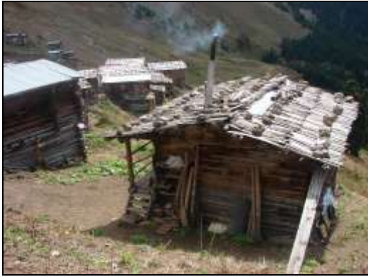
Figure 5. The roofs of plateau houses in the field are slanted in both sideways
