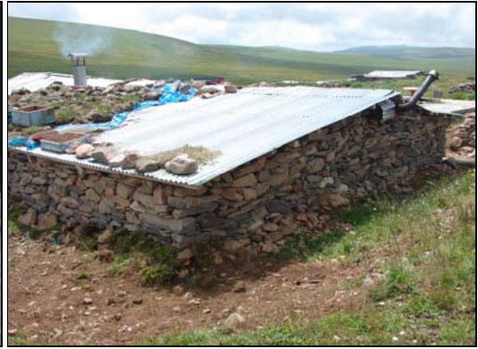
Figure 6. A plateau house which basic building material is stone
