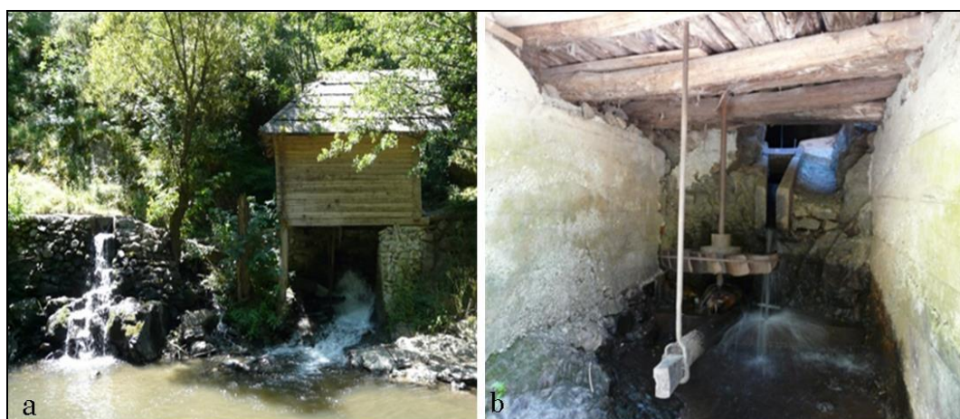
Figure 3. Watermill on Rudăria valley (a); Functioning mechanism of a watermill (watermill wheel - "ciutura") (b)
