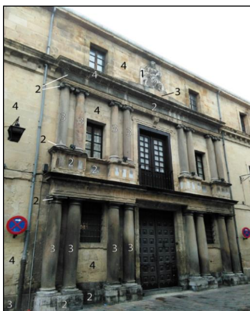
Figure 6. The façade of the old school that later became the Hospicio de San Prudencio, built in 1589, is a good example of the neoclassical style and comprises the main types of stone used in masonry and sculpture in Vitoria-Gasteiz, 1. Paleocene limestone ( Lumaquela de Ajarte ); 2. Upper Cretaceous limestone ( Caliza Negra de Anda ); 3. Albion sandstone ( Arenisca de Sierra Elquea ); 4. Miocene sandstone ( Arenisca tipo Fontecha ).
