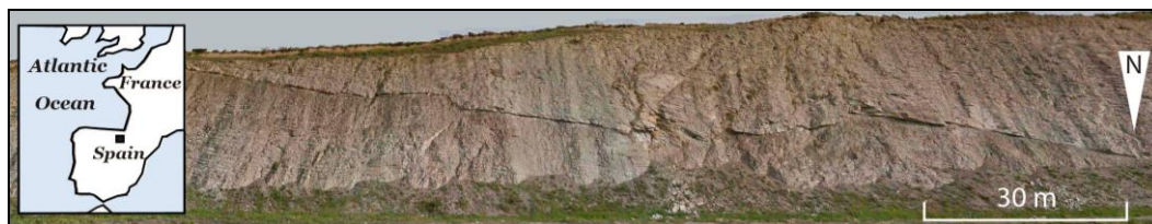
Figure 1. Location of Vitoria-Gasteiz and the slope of highway A-1 (42.827634, - 2.761958), Characteristic Upper Cretaceous marly limestone, The series dips toward the south and shows small sedimentary extensional faults and a gentle angular discordance at the base of the limestone (Overview is from Google Street View. Accessed 13 Dec 2017)
