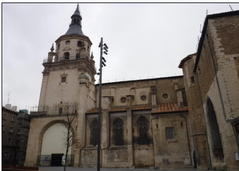
Figure 2. Southern facade of the Cathedral of Santa Maria. The ashlar is composed of Paleocene limestone ( Lumaquelas de Ajarte ). The masonry is Campanian calcarenite ( Calcarenitas de Olárizu )
