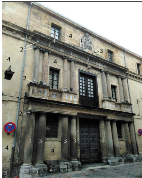
Figure 6. The façade of the old school that later became the Hospicio of San Prudencio, built in 1589, is a good example of the neoclassical style and comprises the main types of stone used in masonry and sculpture in Vitoria-Gasteiz, 1. Paleocene limestone ( Lumaquela de Ajarte ); 2. Upper Cretaceous limestone ( Caliza Negra de Anda ); 3. Albian sandstone ( Arenisca de Sierra Elguea ); 4. Miocene sandstone ( Arenisca tipo Fontecha ).
