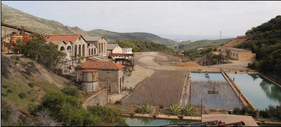
Figure 4. Principe Tomaso washery, Cantiere Piccalinna
