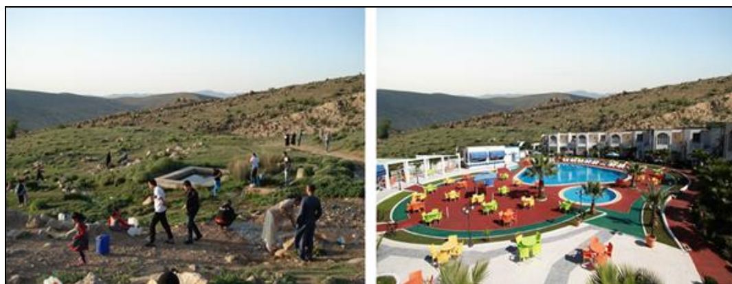
Figure 8. Development of Ain Oucherchar site for the creation of the eco-holiday village
