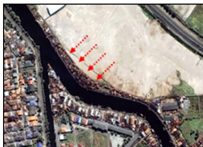
Figure 1. Aerial shot on the location of the fish fumigation industry in Bandarharjo
