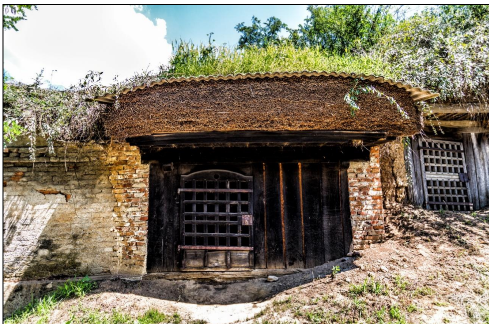
Figure 6. Brick cellar Salacea
