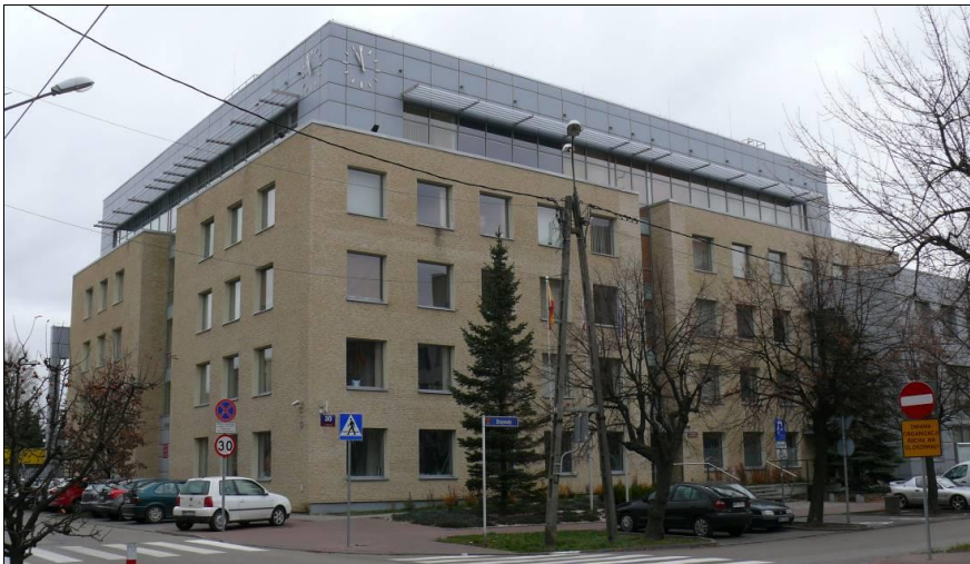
Figure 12. The outer walls of the building of District Authority Office are covered with the elevation brick made of the mixture of natural aggregates: granite, marble and mica
