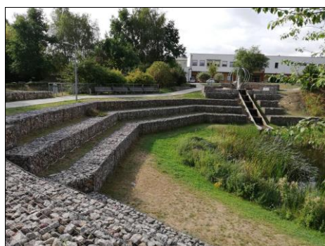
Figure 9. Gabions in the Żwirowisko Park stabilize the slopes of the former gravel pit and have aesthetic and decorative function
