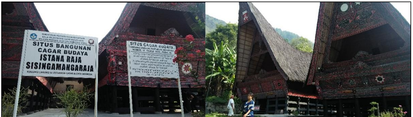
Figure 8. Conservation Aspect Concerning Public Facilities In Istana Sisingamangaraja, Bakkara (Source: Author, 2019)
