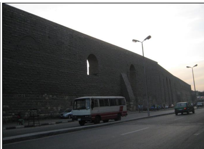
Figure 11. Another view of the aqueduct, showing its height and length
