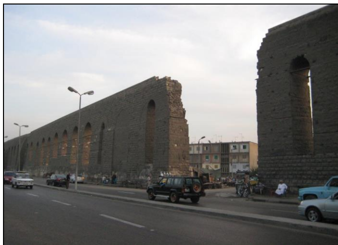
Figure 10. The Magra El Eyoon Aqueduct
