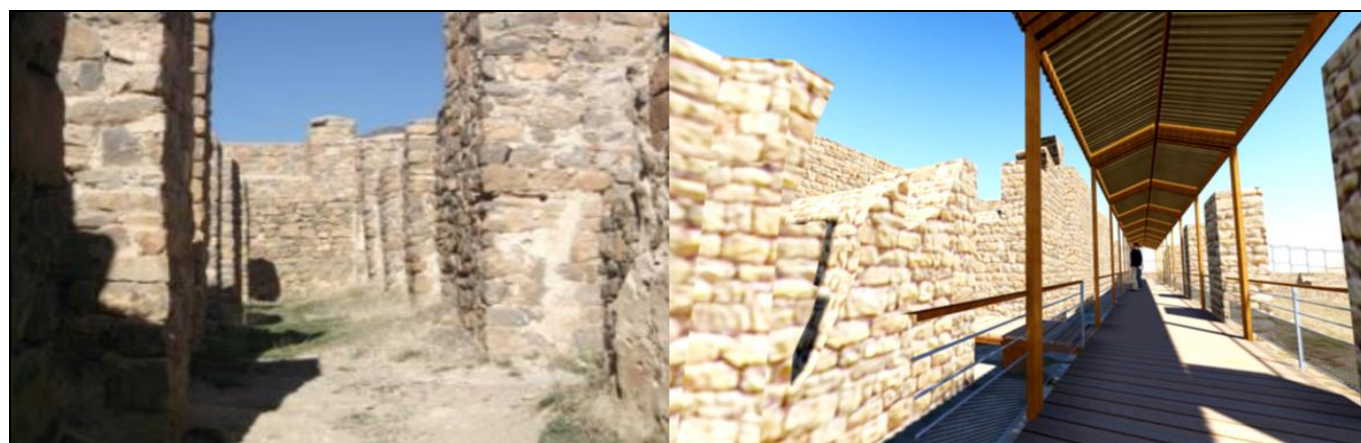
Figure 8. Intervention involving the construction of a protective roof on the Al Manar palace (authors)
