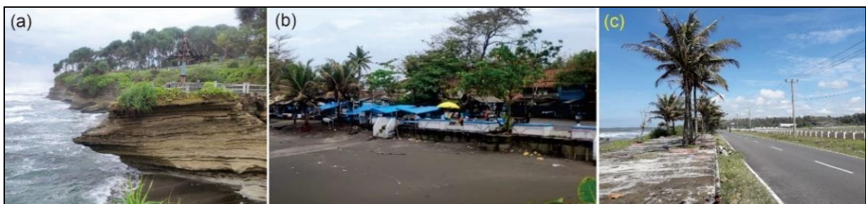
Figure 9. The appearance of some physical and human parameters in Class 4 The rock cliff icon of Batu Hiu, (b) The semi-permanent structures in Batu Hiu's dunes, (c) The pedestrian and buffer zone near Legok Jawa (Source: Author, 2022)
