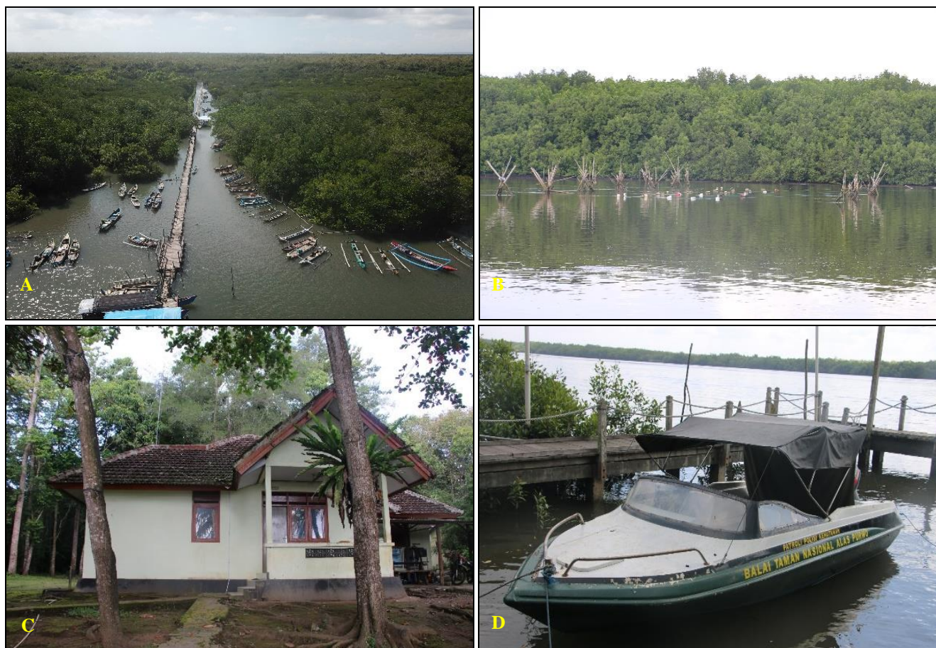
Figure 10. The condition of the main pier, Segara Anakan for fishing, resort and boat parking area for forestry police patrols (A – D) (Source: Author, 2022)
