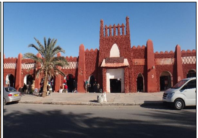
Figure 3. Local architectural character - Adrar city center
