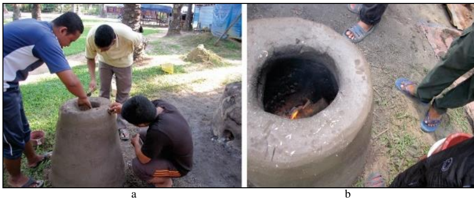
Figure 4. The process of attaching the tuyere to the furnace wall to complete the shape of the built furnace (a) and when the furnace is dry, it is burned to strengthen of the furnace structure (b) (Source: Research data analysis, 2023)
