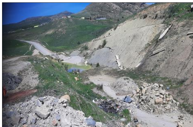
Figure 7. National Road 78 (Setif – Bougaa), section abandoned at Takoka, due to landslide (Source: Authors, 2021)
