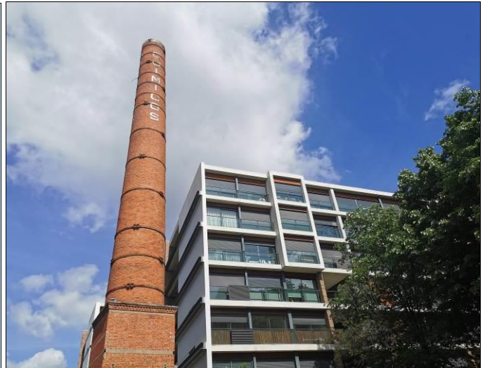
Figure 3. Dismissed chimney in a new residential complex (Source: Authors)
