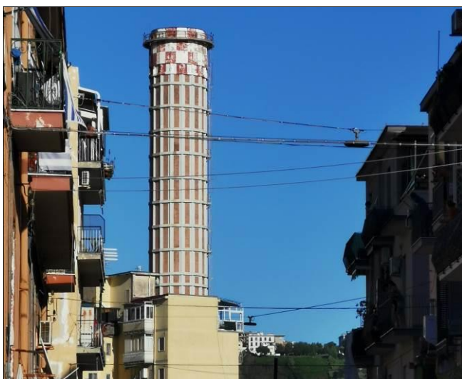
Figure 10. Dismissed chimney (Source: Authors)
