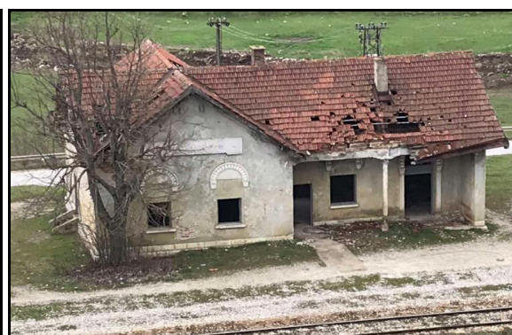
Figure 14. The train station in Dobroshec (Source: own study)
