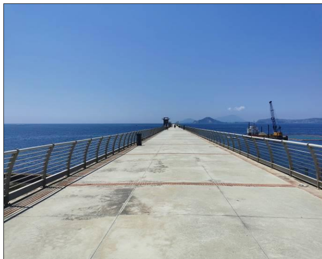
Figure 11. The north jetty (Source: Authors)
