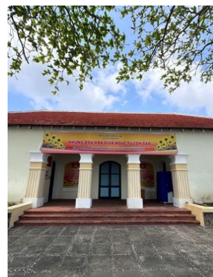
D9 – Former Communal Hall
