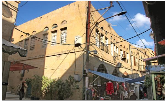
Figure 18. The Abu Alouf Building, Al-Hammam Street: mixed-use building in local yellow limestone construction (Source: Authors)
