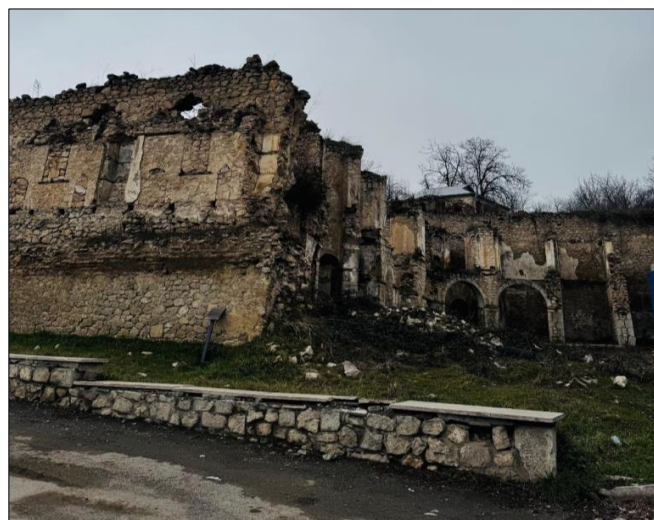
Figure 6. Caravanserai of the Safarov brothers destroyed in Shusha city during the occupation (1992–2020) (Source: The author)
