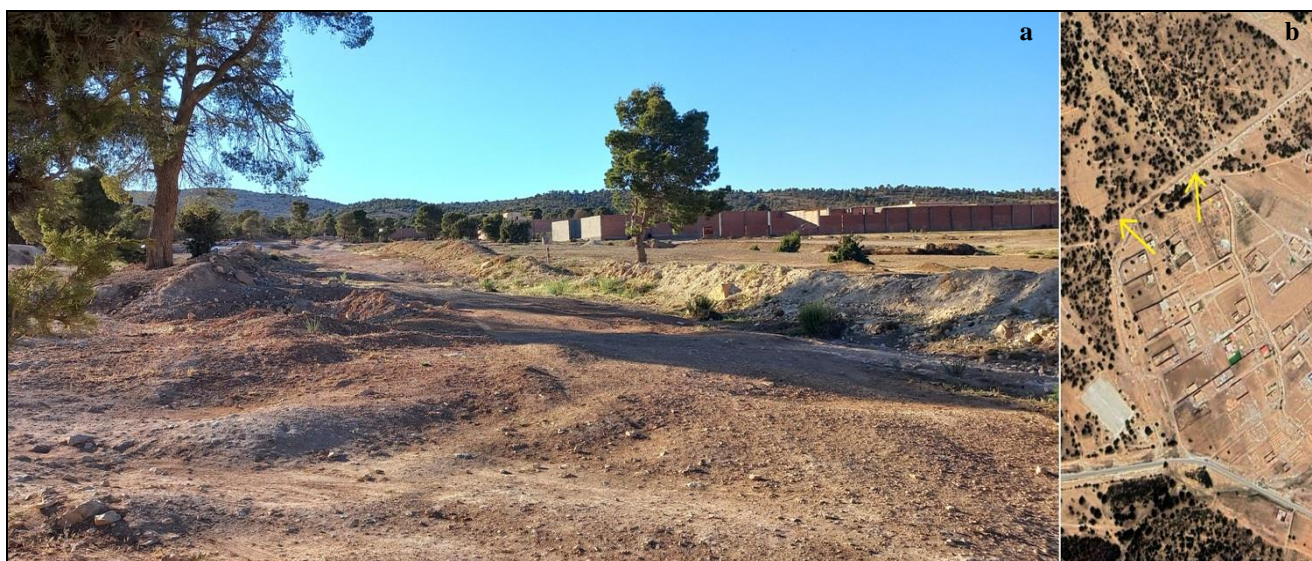
Figure 17. Construction progress towards Senelba Forest (Source: 17a: Authors, 2023; 17b: Googlemaps, 2023)
