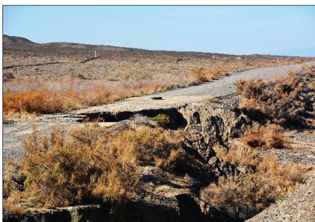
c) destruction of the roadway surface caused by a recent mudflow (monitoring site 9)
